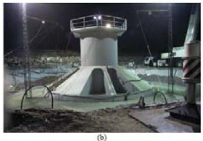
Figure 13. Installation of the prototype foundation at the test site in Frederikshavn: (a) during installation, (b) at the end of installation.
