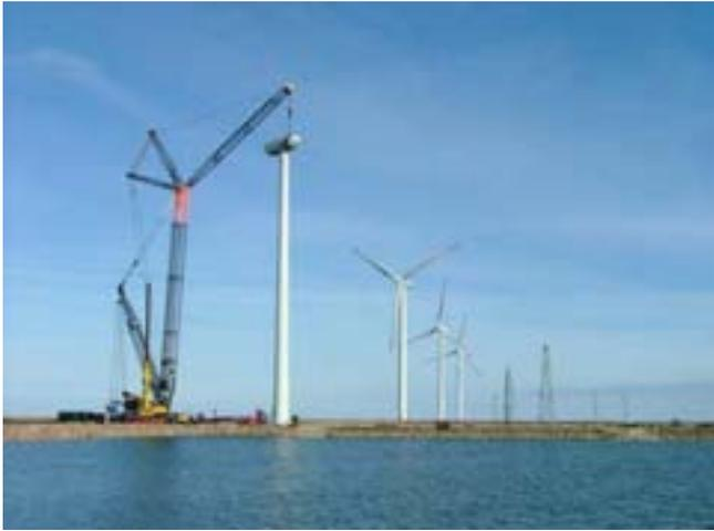
**Figure 19. Replacement of nacelle in the spring 2005. The four wind turbine at the test field in Frederikshavn is shown. The Setup for combined loading of 2x2m bucket is also shown.**
