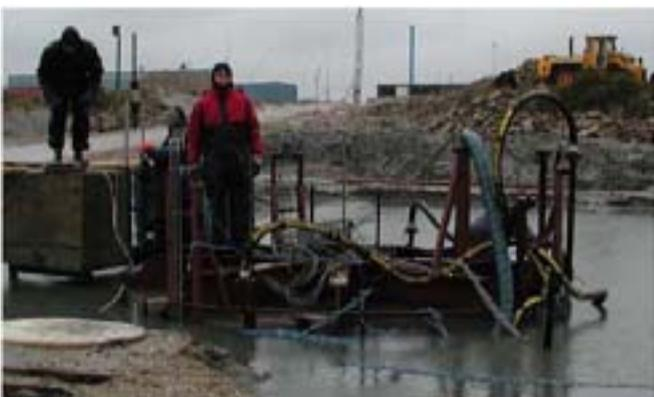
Figure 12. The 4x4m bucket successfully installed.
