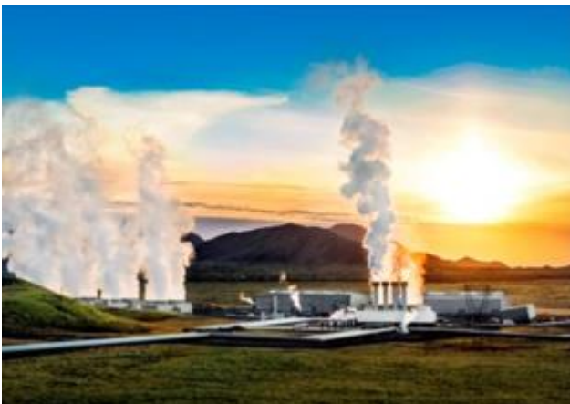
Photo from powerplant website showing an overview of the plant.
