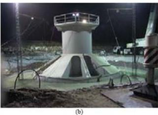
Figure 13. Installation of the prototype foundation at the test site in Frederikshavn: (a) during installation, (b) at the end of installation.
