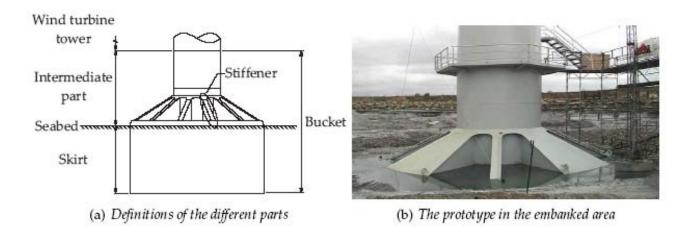
Figure 2 Definitions and illustration of the prototype of the bucket foundation in Frederikshavn.
