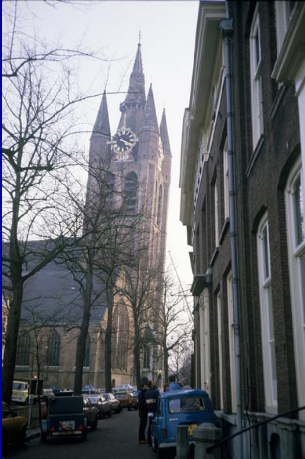
Differential settlement Delft
