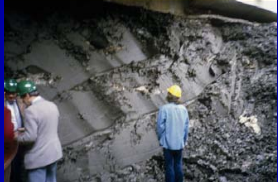
Inspecting London Clay in deep excavation
