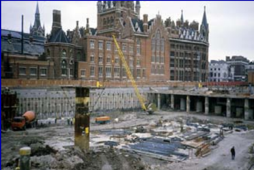
Deep excavation for British Library King's Cross, London
